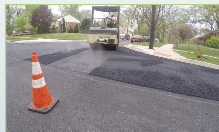
New asphalt is placed and compacted
